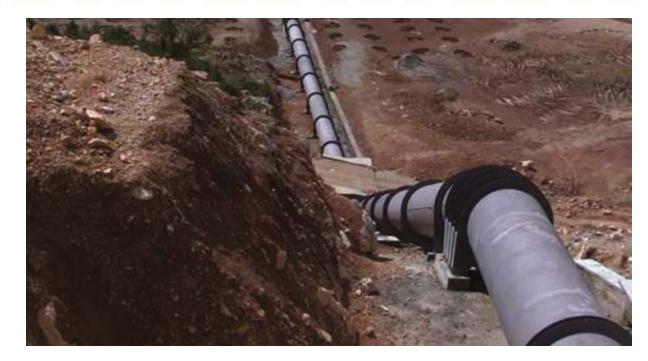
Sewerage lines comprise pipes and channels that transport wastewater and stormwater from residential and industrial areas. Pipes used in these systems are typically made from concrete, reinforced concrete, high-density polyethylene, PVC, or corrugated plastic. In sewer lines the flow rate of wastewater must be higher than the minimum value identified in the technical specifications. This prevents the settlement and accumulation of debris in pipes.
